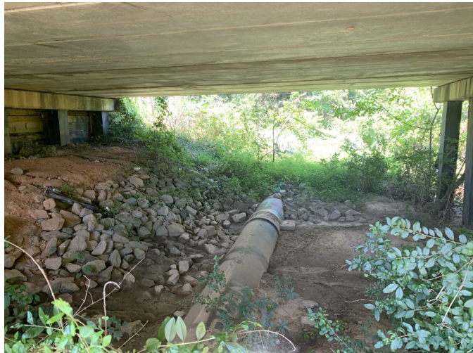
Sewer line under W Balfour Ave bridge
