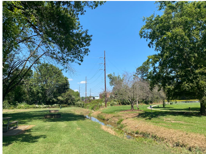
Transmission Lines along Hasketts Creek
