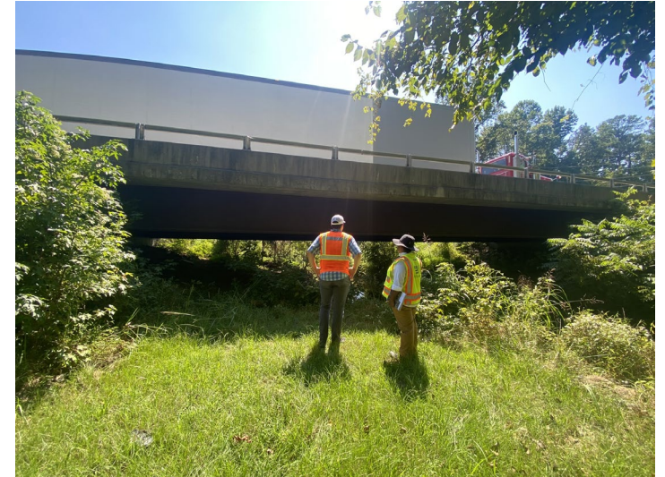
W Central Ave bridge at Hasketts Creek
