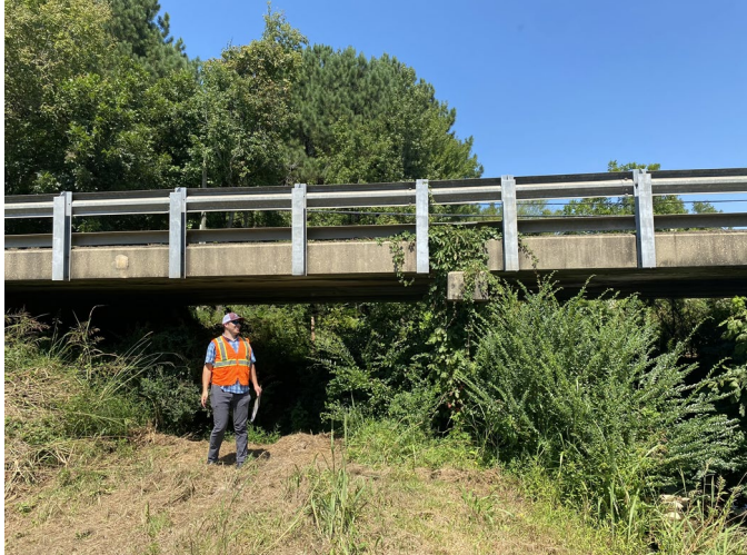
W Balfour Ave bridge at Hasketts Creek
