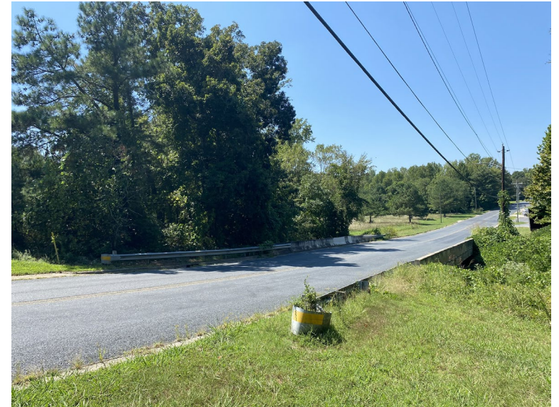
W Bailey Street bridge over Hasketts Creek
